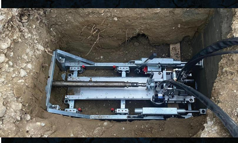
For use in the excavation pit, the MiniRockDrill, including pit frame, can be quickly placed as a complete drilling rig with an excavator. If no lifting gear is available, the pit frame, the drill frame and the rotation gearbox can be installed individually by hand. With the integrated hydraulic hand pump and the two cylinders on the pit frame, a quick fixation is guaranteed and it can be quickly retensioned during operation if the frame becomes unstable.
